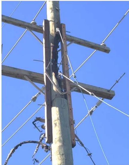
Restore before repair example
